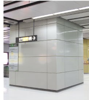
Aluminum veneer external corner installation sample / 铝单板外部转角安装实例
